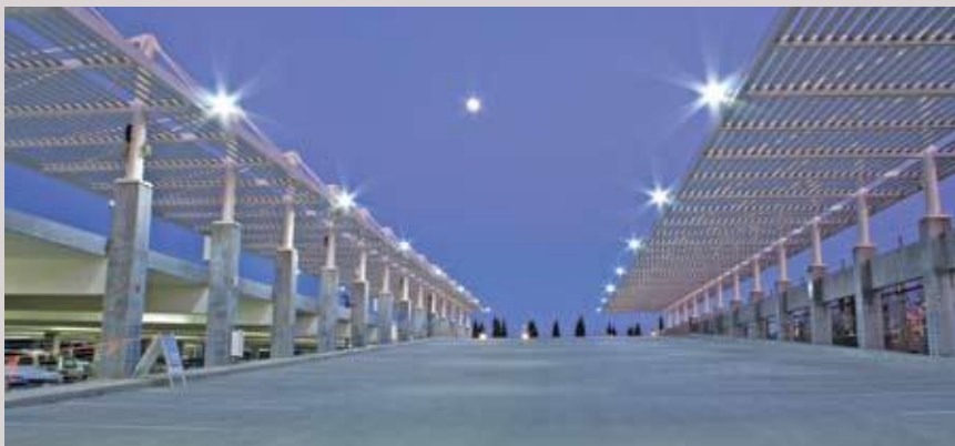
The lighting in the parking structures at UC Davis provided an opportunity to implement cutting edge technology.
